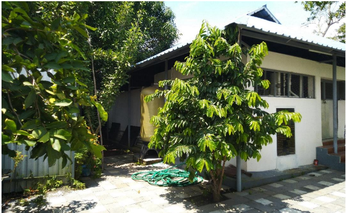
Common Sewage Treatment Plant (STP) for houseboats at Kavanattinkara, Kumarkom
