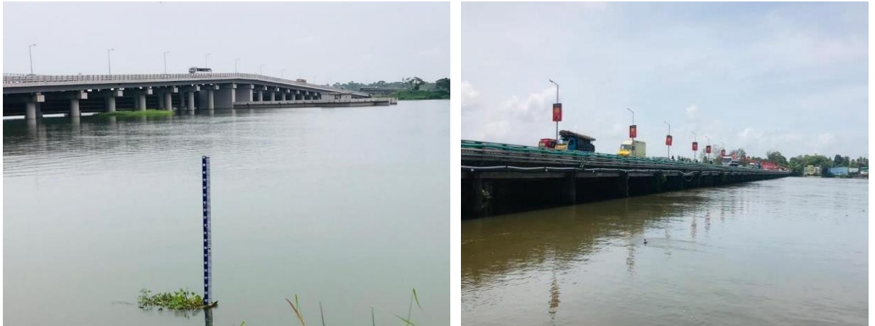
Thanneermukkom Barrage and Thottappally Spillway 45
